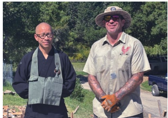
Below right: Hojo-san and Eric Scudder of River Town Electric in Petaluma. Eric has donated his electrical work for the Kanzeon House and the Sanmon Mountain Gate
