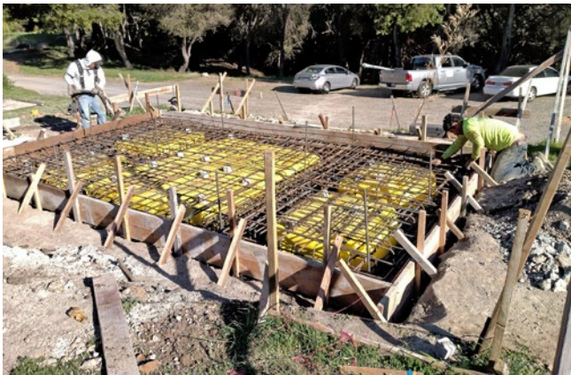
Far left: Preliminary foundation work for Sanmon Gate
